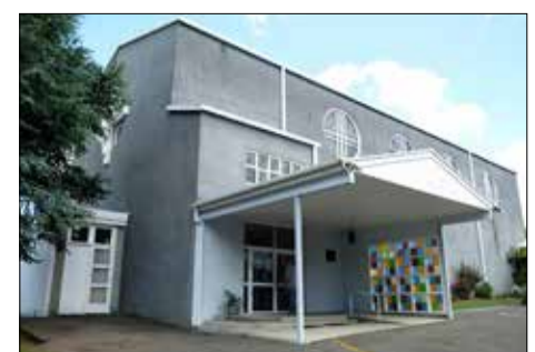
St Mary's Church, Taihape – a modern historic building.
