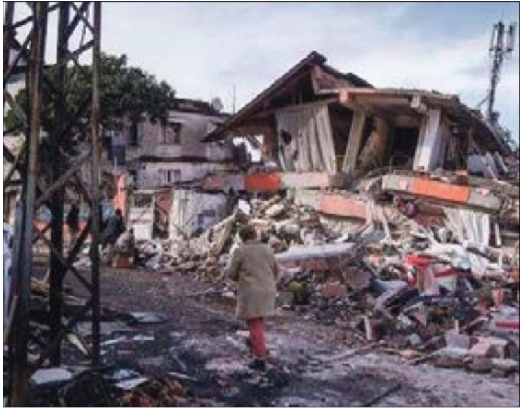
Buildings demolished by the earthquake in Antioch.
