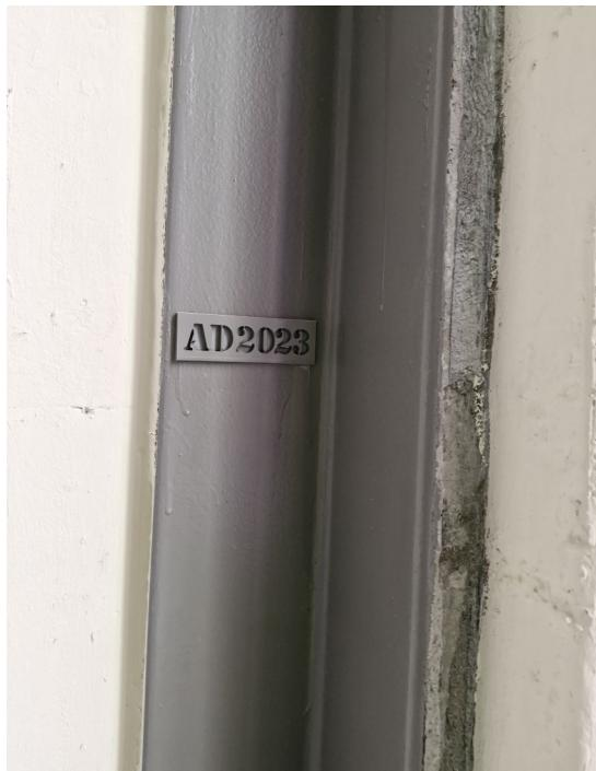
Cathedral earthquake strengthening beam that reads **AD2023**, which is the year this strengthening beam was installed. A lot of work has gone into making the building safe for us now and for the future.
